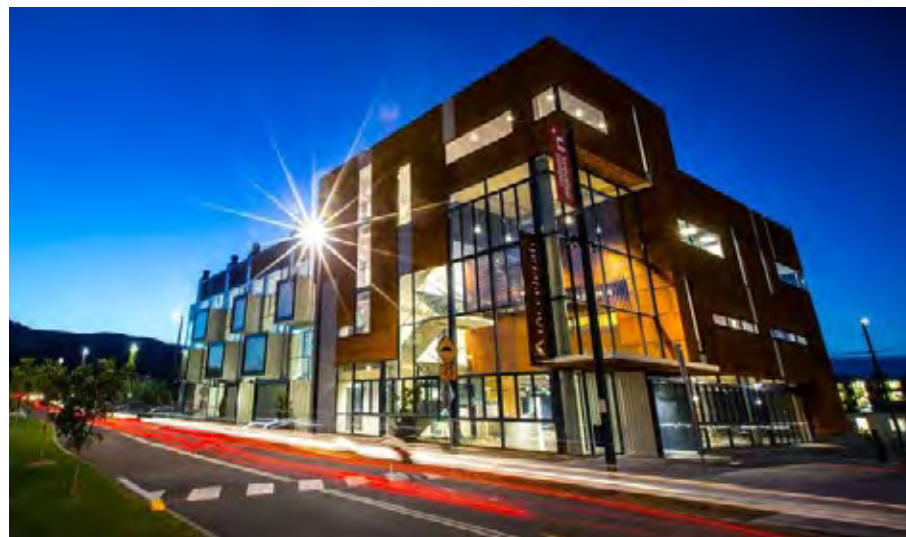
Institute for Superconducting & Electronic Materials (UOW)
